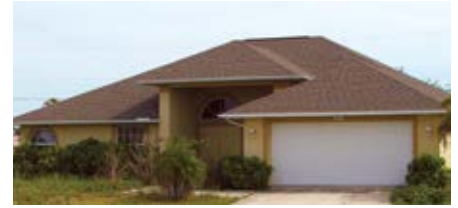
This home is classified as Hip if all four elevations look similar to this.
