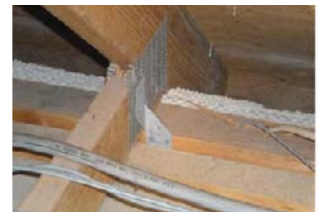
This photo shows clips as the roof to wall attachment.
